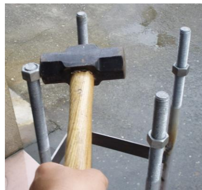
Place the nut and adjust pole with mallet
