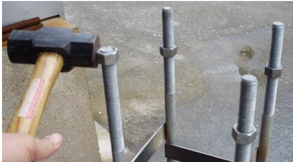
Place the nut and adjust pole with mallet
