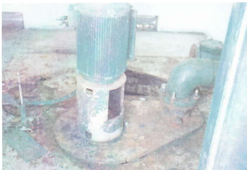
Photo 6: Sewage pump motor – poor state of repair
