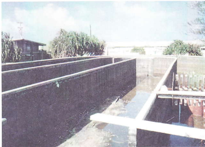
Photo 3: Empty basin showing grit buildup
