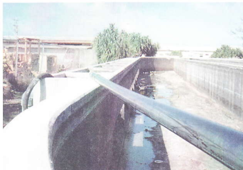
Photo 2: Empty basin showing grit buildup
