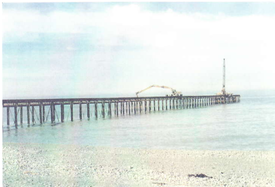
Photo 10: Outfall construction using pile platform
