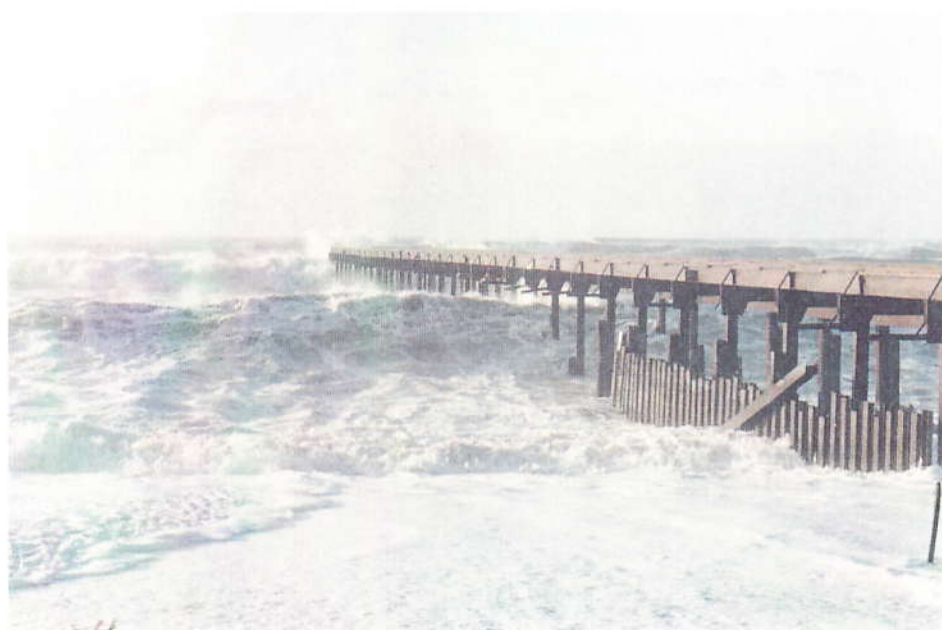
Photo 12: Piled platform showing wave tolerance
