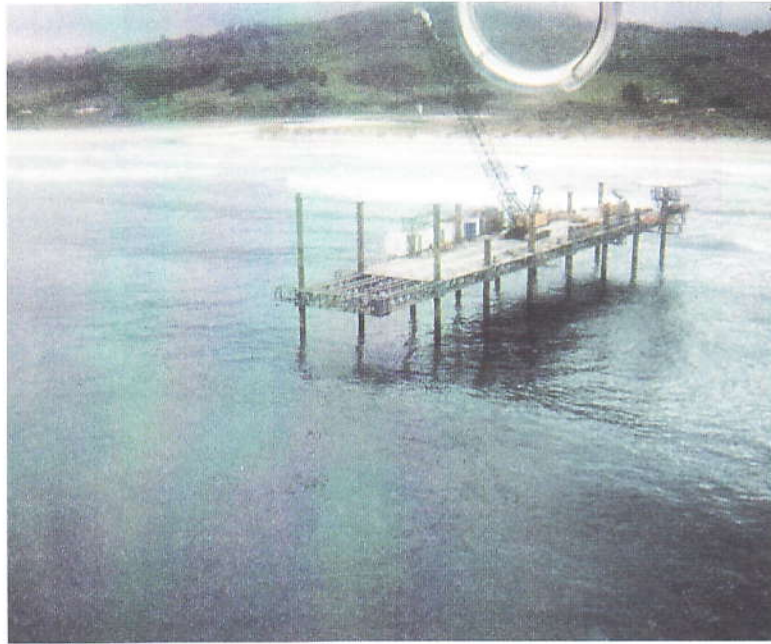
Photo 9: Outfall construction using jacking platform
